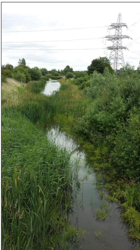
Examples of natural environmental features at National Grid's Thorpe Marsh substation.
